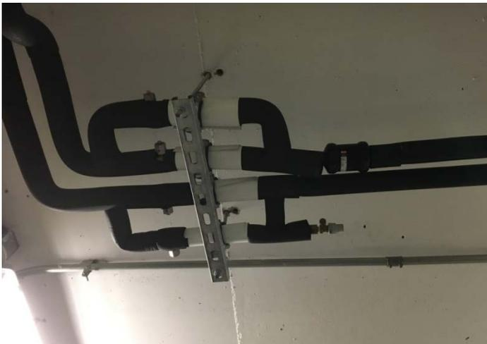
Figure 4 Filter and bypass / NRV assembly
