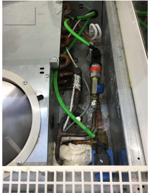
Figure 2 EEV installation
