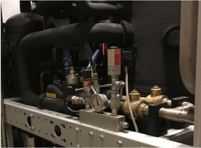
Figure 1 Parallel high pressure valves
