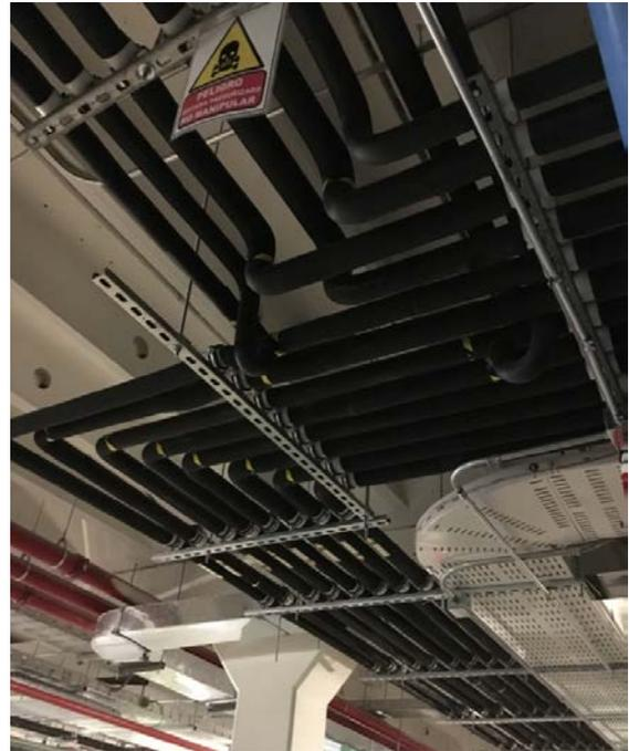
Figure 6 Pipe support and insulation
