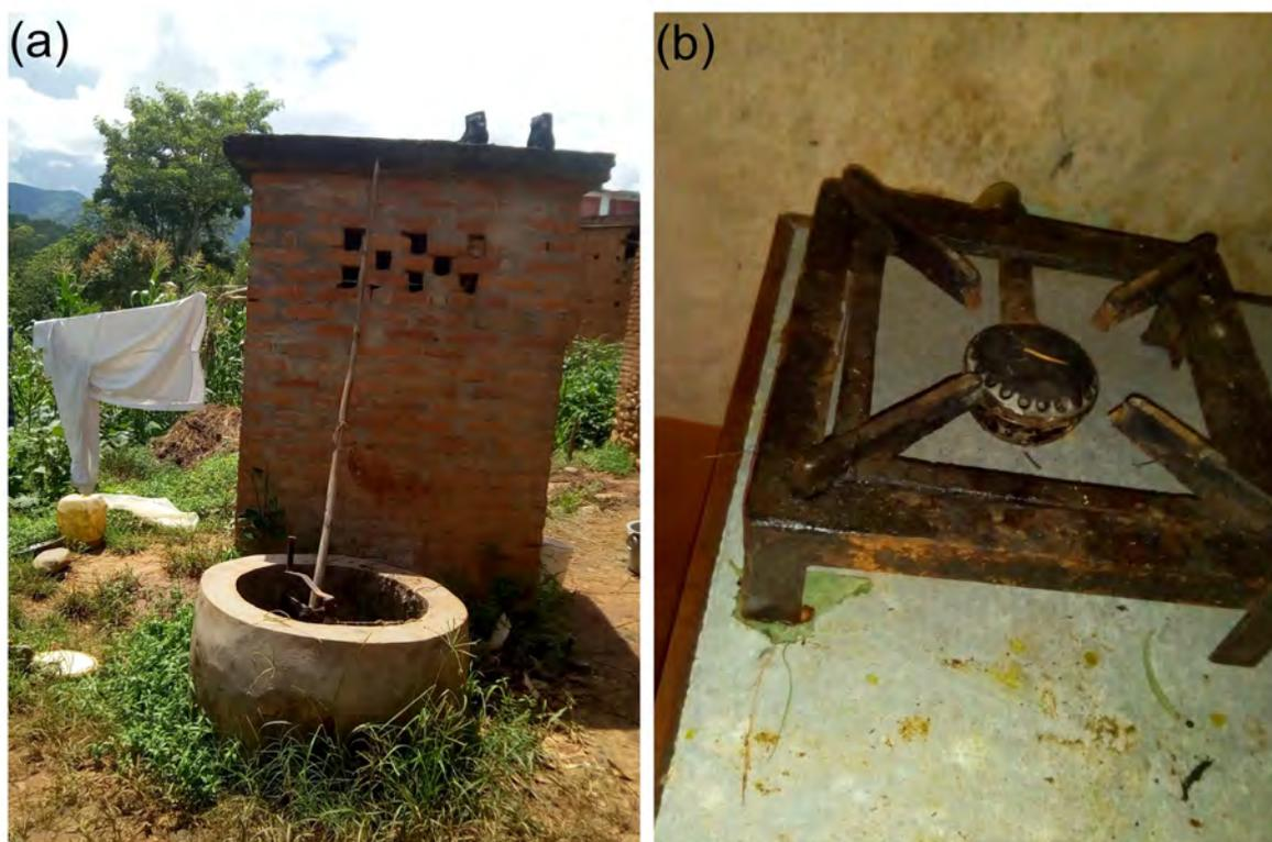
**Figure 1.** Biogas system components. (a) The cement ring is the mixing chamber (with a hand-crank steel mixer) for adding fuel to the digester. The latrine, behind the mixing chamber feeds directly into the digester. (b) A typical biogas stove burner.
