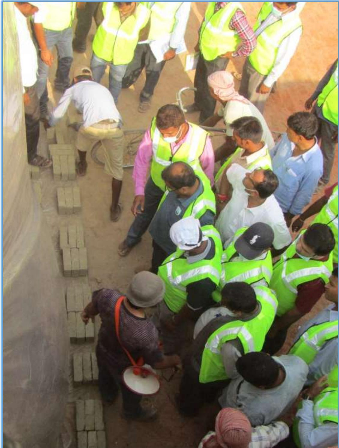
Photograph 4: Practical demonstration of zigzag stacking
